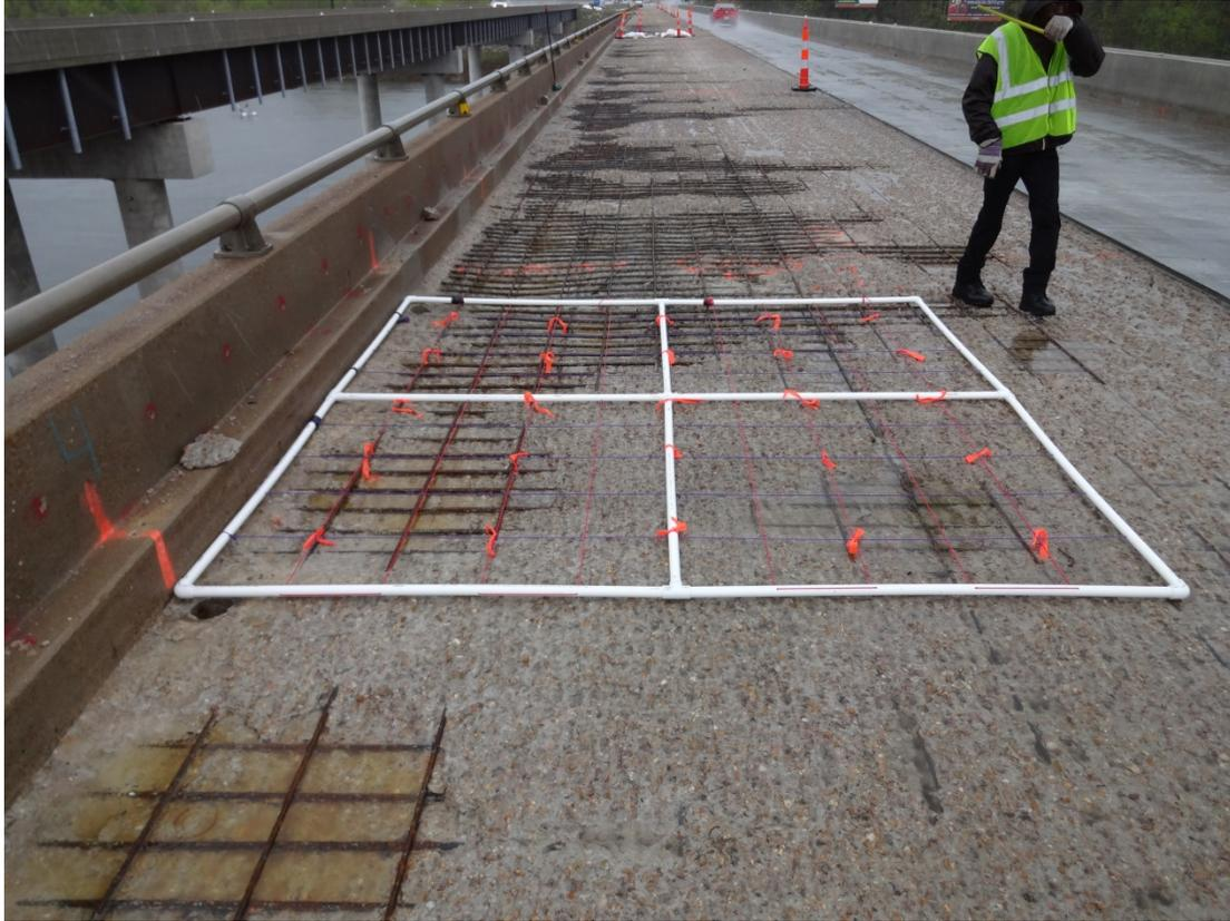
**Figure 15: The Bridge Deck Surface after Conducted Hydro-demolition Test.**
