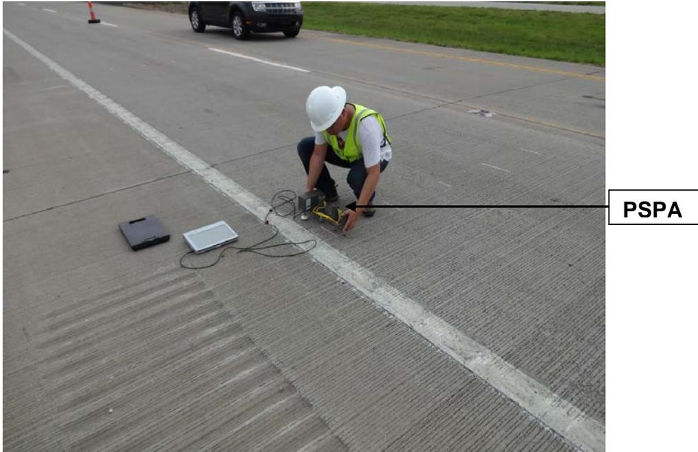
**Figure 08: PSPA Data Collection in the Field for Pavement Evaluation.**
